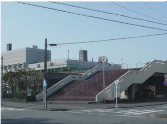
Fig. 5. Practical tsunami mitigation from Japan to permit the populace to climb to the roof of the buildings in case of warning for a nearby source of tsunami [5].
