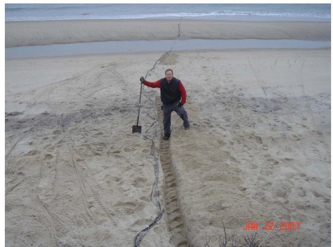
Fig. 7 Trenching MAVS cables across the beach. Sandbar is visible offshore.
